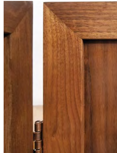
Close-up of C molding with mitered corner on floor screen
