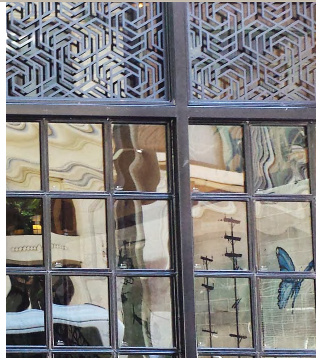
Delta General Contracting, Little Sister storefront, Tarzana, CA; ¼" Outdoor MDF, Hexagon Puzzle Pattern
